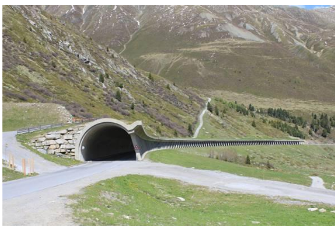
Figure 1.9: Road protection against avalanches in the Sellrain valley, Tyrol, Austria. Source: H. Cammerer.
